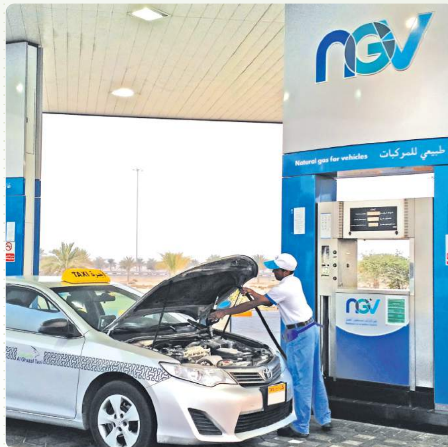
CNG pumps at an ADNOC station
