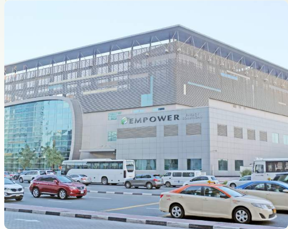
Empower's district cooling station, Dubai
