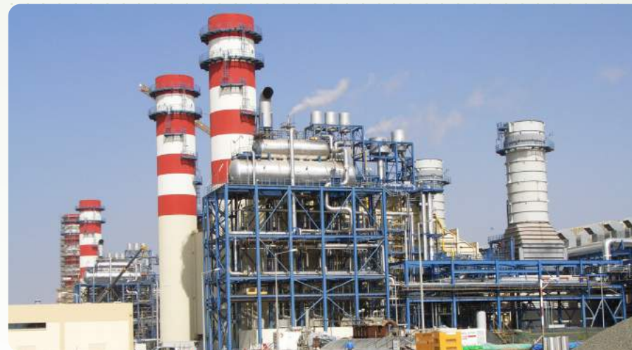
A combined cycle power plant, Abu Dhabi
