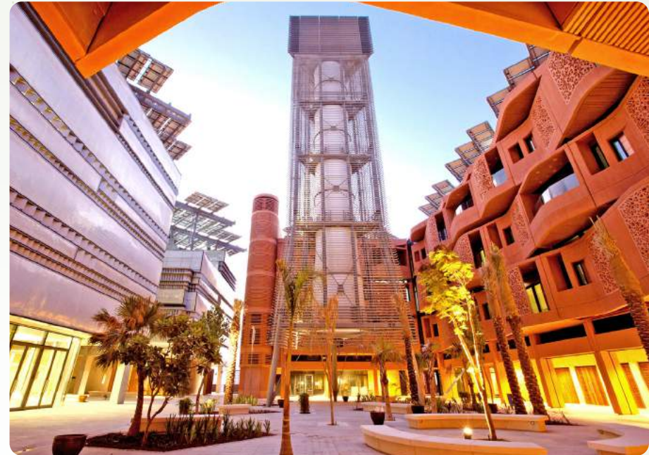
Masdar City and a wind tower for cooling
