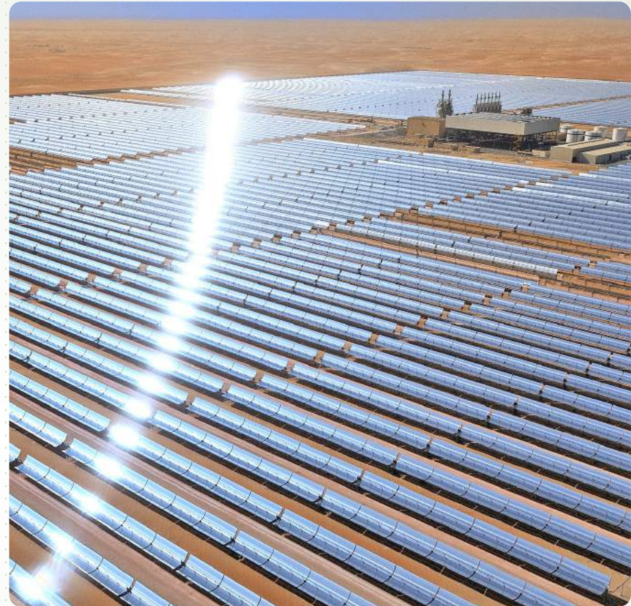
Shams 1 CSP plant
