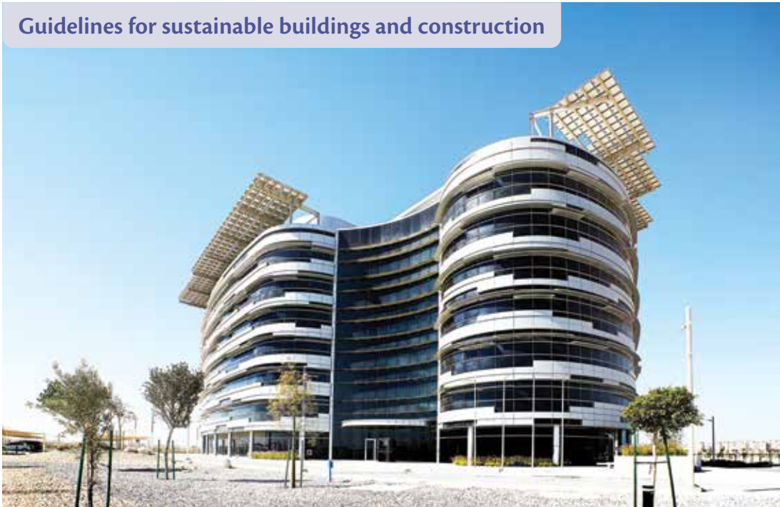
IRENA headquarters building in Masdar City, which was the first building to obtain a four-pearl rating under the Estidama scheme
